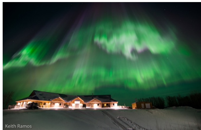
Yukon Koyukuk Elder Assisted Living Facility
